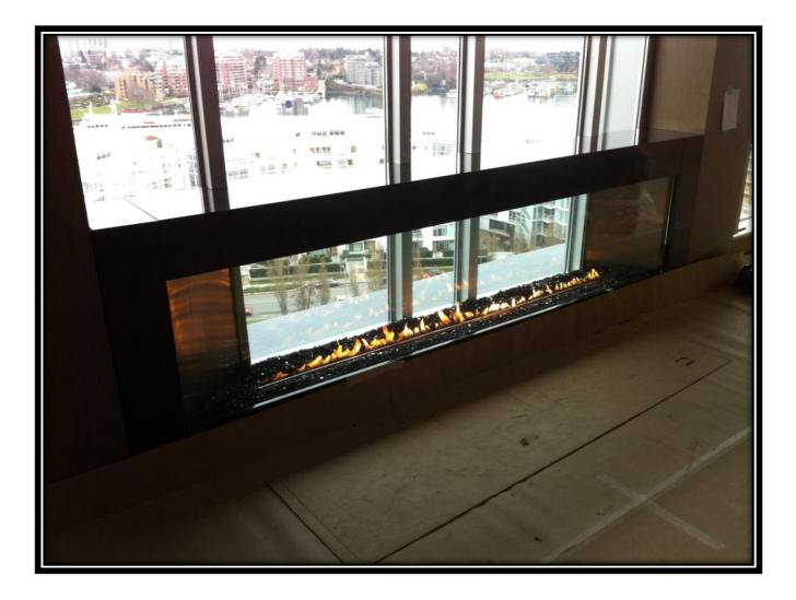
8ft wide and 3ft deep this see through was installed at 9000ft on propane.
