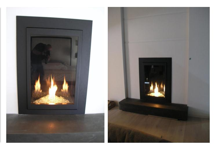
One of our early custom units, we had to deal with a lot of combustibles around the unit. This required some out the box thinking and technology borrowed from our production unit LE with patented insulation technology.
